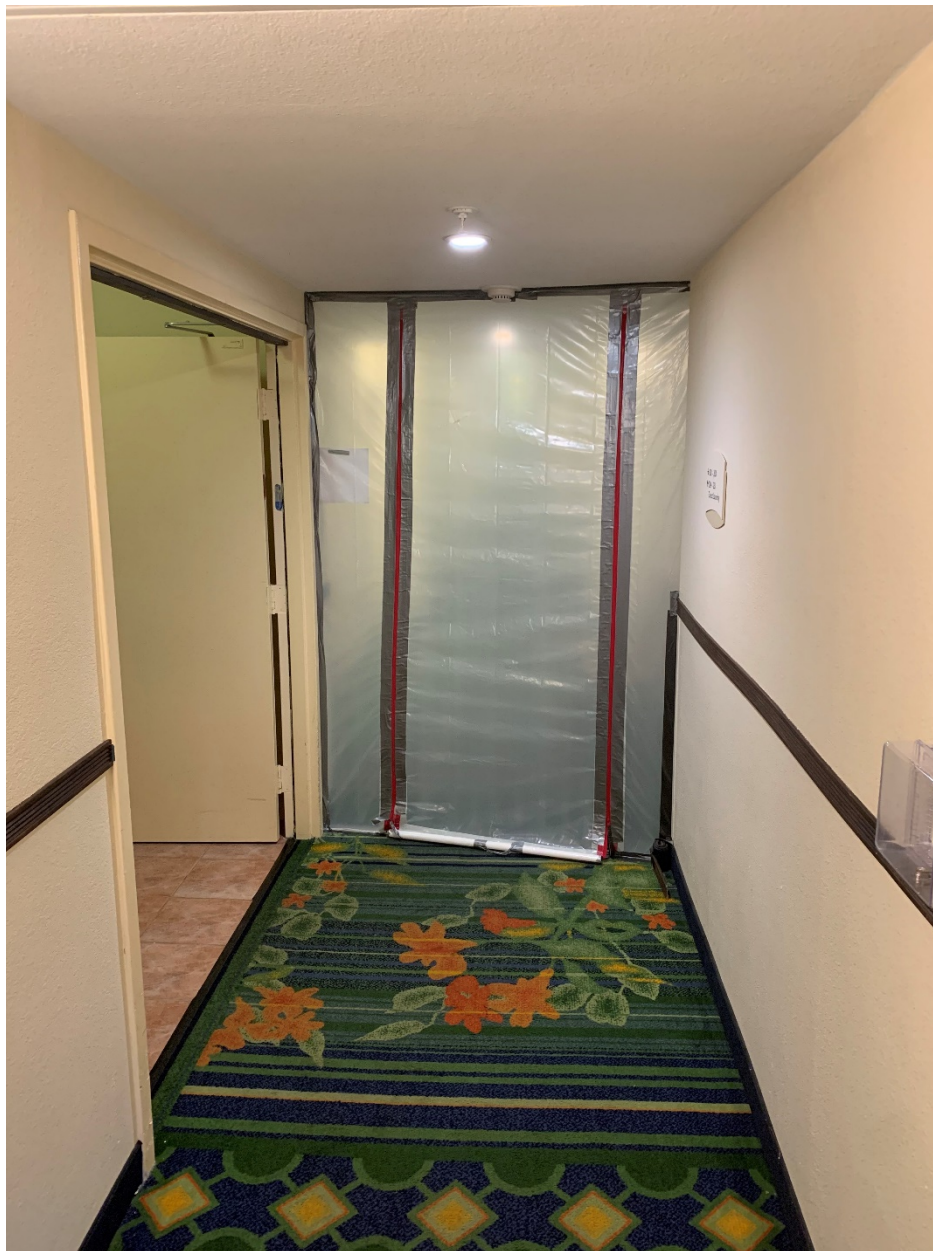
Figure 3: Sample Plastic Barrier to Isolation Zone Area
